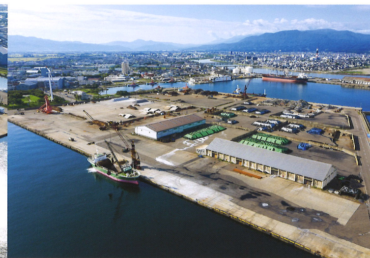
中央埠頭(鉱産品・木材岸壁) 北側に鉱産品岸壁、南側に木材岸壁があり、直江津港における主要な岸壁となっております。木材岸壁の係留能力はD/W15,000t、鉱産品岸壁はD/W50,000tの能力があり、直江津港で最大の係留施設です。 Center pier (Kohsanhin & Lumber berth) It is a main berth at Naoetsu port and there are Kohsanhin berth on the north side and Lumber berth on the south side. Lumber berth has a mooring ability of D/W 15,000t and Kohsanhin berth has a mooring ability of D/W 50,000 which is the biggest mooring facilities in Naoetsu port.
